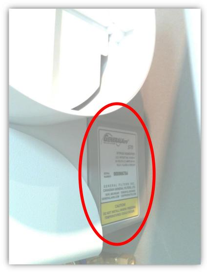
The model and serial numbers for these models can be found on the side of the humidifier, on a yellow and white sticker. This area of the humidifier is also called the "chassis".
